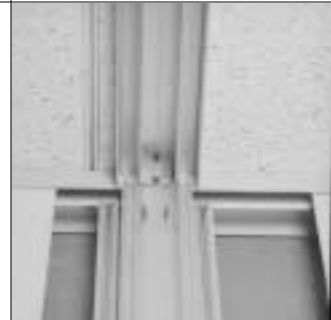
Secure intersecting ceiling runners with angle clip. Angle clip with longer leg can also be used to secure the stud assembly in the proper position.
