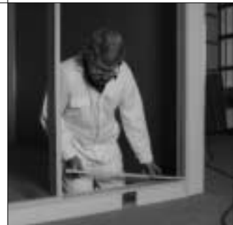
27. ...and secured to sill.
