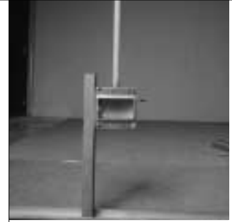
3. A vertical piece of strut runner can be used to support electrical boxes.
