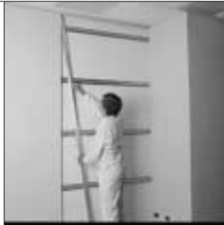
11. Vertical furring splines are positioned . . .
