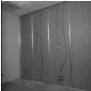
7. Flexible prewired electrical systems can also be used in ULTRAWALL partition systems. Photo illustrates one side of wall erected with T-studs prior to electrification.
