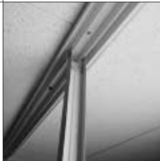
Method 4. Slit strut at its flange/web corners and fold web down. Strut flanges will overlap aluminum inner legs.
