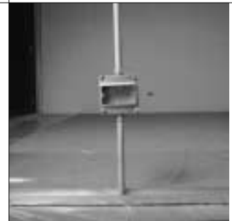
6. A piece of conduit can be coupled to the electrical box for support.
