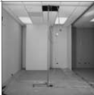
8. Flexible prewired electrical components can also be installed through ceiling runner prior to erecting any panels..
