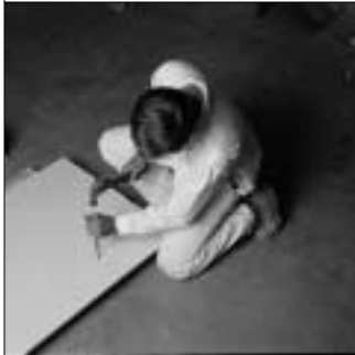
22. Wall board saw is used to easily cut required opening.
