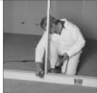
21. ...and screw-attach top and bottom.
