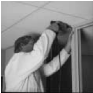
11. Strike jamb must be positioned to ensure proper door closure and securely fastened.
