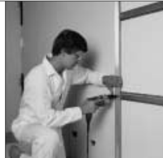
12. . . . and screw-attached to horizontal furring members.
