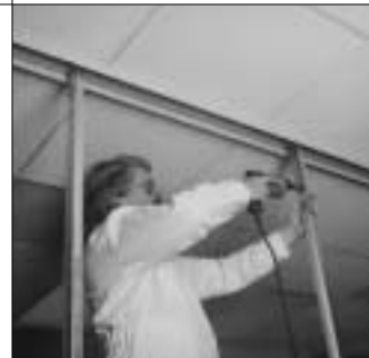
Method 5. Engage strut runner to stud extension and screw-attach through pre-punched holes in extension.
