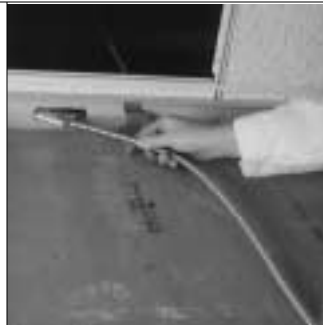
10. ...and mating hole in ceiling tile.
