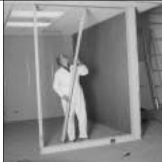
20. Position glazing rail plumb and square...
