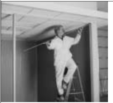
16. Large glass openings divided by vertical mullions require continuous AGL-341 glazing cover to be snapped into ceiling runner.
