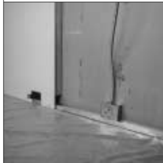
13. ...and routed to box at floor.
