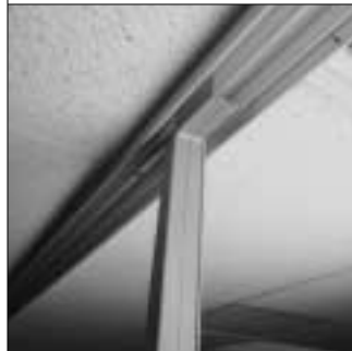
Method 3. Cut and bend strut runner to overlap strut legs and inner flanges of ceiling runner. Screw-attach strut to ceiling runner at corners.
