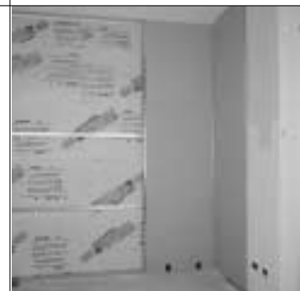
18. Supplemental horizontal members angle clipped to T-studs are required for partition rigidity.
